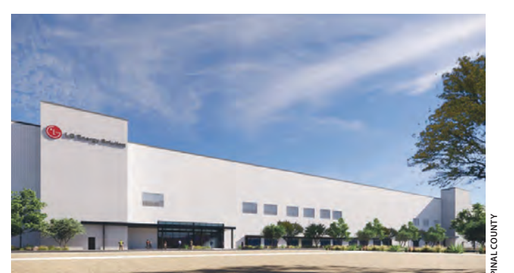
LG Energy Solutions Arizona is expected to break ground on a battery manufacturing complex in Queen Creek, Pinal County, in the first quarter of 2024. The project represents $5.5 billion in capital investment, 278,709 square meters of space, and 3,700 new jobs.
